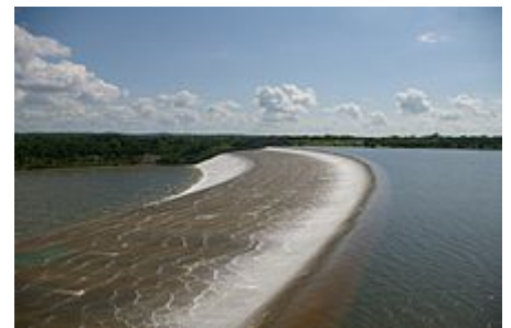
Water going over emergency spillway for the third time in the dam's history July, 2007
